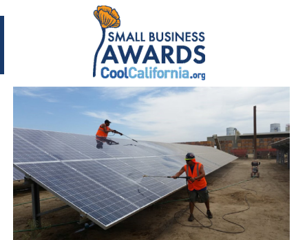
Mr. Squeegee's team cleaning a solar panel array in an agriculture community.
