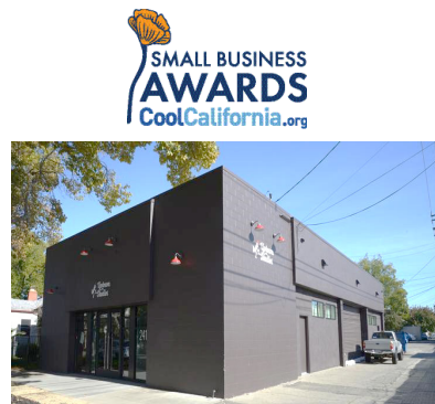
Uptown Studios converted an old warehouse space into a modern, energy efficient workplace.
